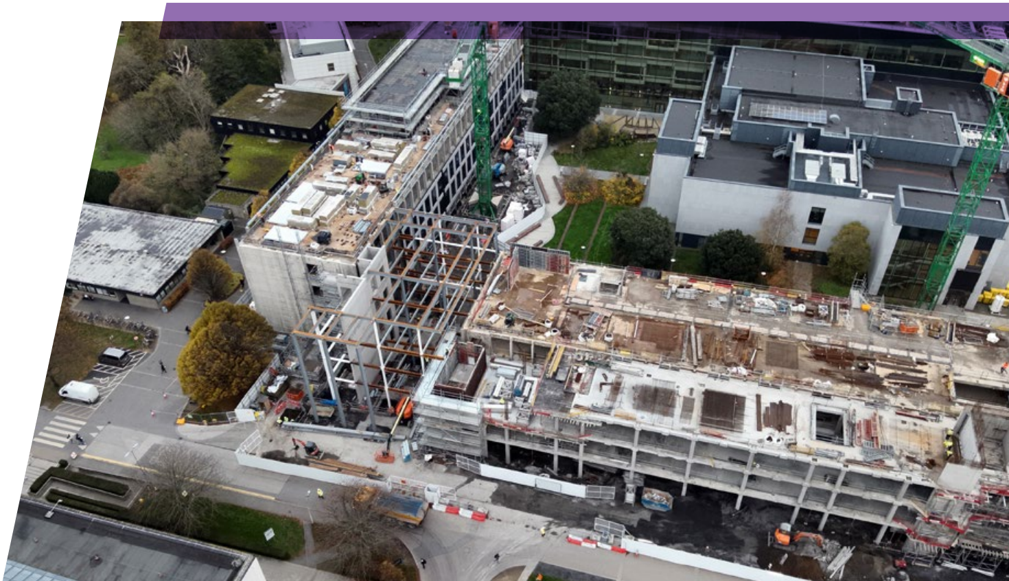
Renovation works continue on Science Phase 3.
